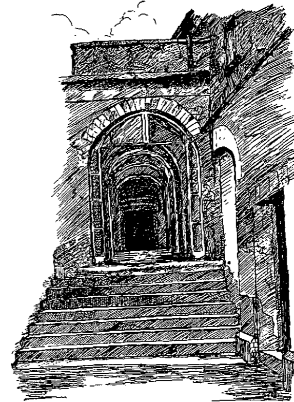
THE PASSAGE TO THE NEW LABORATORIES.
